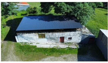
this has had a steel structure built over with box profile clad roof.
